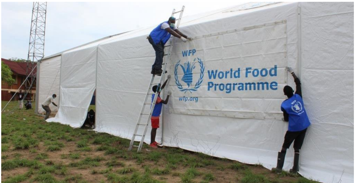
WFP's Logistics team constructing the mobile storage unit. Photo: WFP/John Monibah
